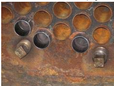
New tubes have been fitted and expanded
