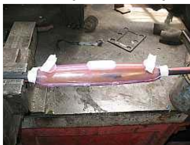
L02 – A professional looking epoxy filled cable splice for the new coach's ground power DB.
