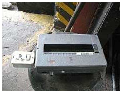
L03 – A stripped and cleaned distribution board prepared to be mounted in the old running shed. We are rigging the shed up to supply head-end-power, to be able to power up a parked train without having to start the generator.
