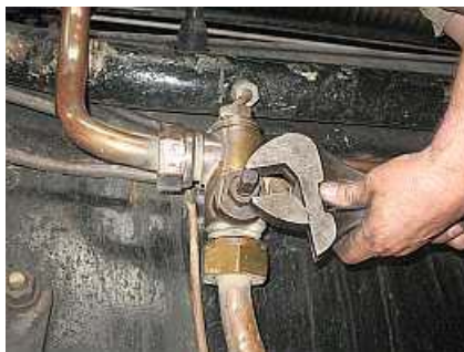
G01 A close up of the Class 15CA No.2056 Drifter Valve with Johann adjusting his wrench to fit the gland packing nut. The cab is to the left of the picture.
