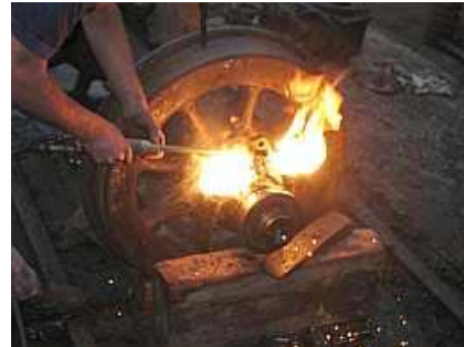
A09 ☞ Inelegant defeat ☞ using a torch to cut up a bearing after it cannot be withdrawn from the shaft. The flames are from the residual degreaser and diesel fuel that has ignited.
