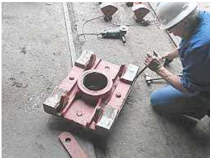
B10 Fred Sewell is levering off the two strip bearing plates from the Bolster plate. (Upside down) This pic also shows the ramps in the corners that engage the large quadrants of the swing links
