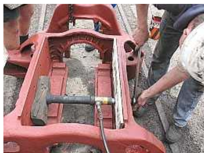
B14 An overhead view of the hydraulic jack and the spacer arrangement with a span bolt sleeve in the center. This shot was taken before we used a nut between the hydraulic ram and the bolt to drift the
