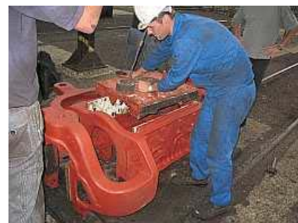
B15 Test Fit. The Bolster Plate is hoisted into place between the slide bearings. It fits between the sides of the Bissel Truck frame.
