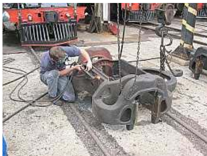
B01 ☞ Shaun Ackerman (☞Smudge☞) tackles the first row of rusty rivets holding the original plate type bolster slide bearings in place. That acetylene torch was in use for Bissel and Axle work throughout the entire day!
