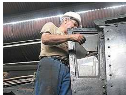
G03 The train was stoned on a recent trip and one of the rocks smashed the fireman's window. Here the frame containing the broken glass is being removed.
