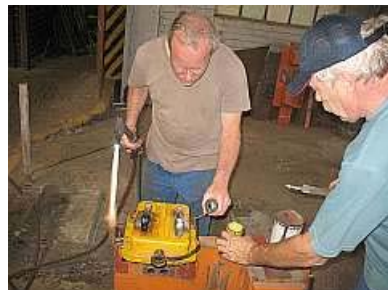
C02 - The generator radiator expansion tank receives some soldering on the flank panels. The tank is poorly designed as the flank panels flex when the water-cooled system is pressurized, contributing to metal fatigue and eventual leaks.
