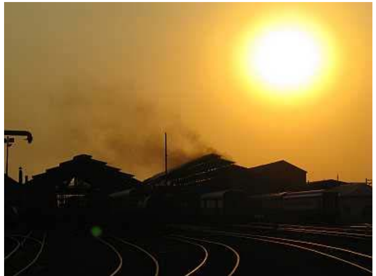
FP14 - Well into the sunset years of steam, 16 years after steam operations officially ceased at the Germiston Steam Locomotive Depot, the old cantilevered running shed roof still emits clouds of evocative coal smoke. Steam is still alive here.
