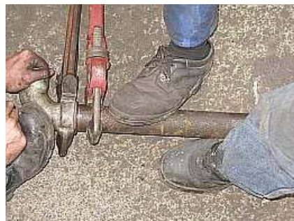
B09 Three men and a baby, or a pipe, in this case. There are two Stilson wrenches in use here so we needed a combination downwards force and sideways restraint.
