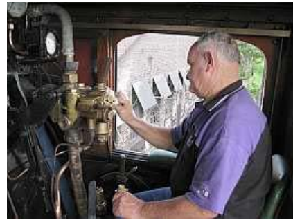
E21 Oom Attie finishes the overhaul with some steel wool n Brass. You can clearly see the incoming steam pipe coming in from top left, neatly wrapped in an insulative bandage. The instrument right behind the pipe is the awkwardly placed speedometer.
