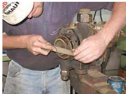
E06 Dressing the sealing surfaces of the vacuum pipe union. This is the face on which the gasket would bear.
