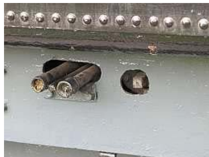
F12 The oil lines for the Stoker Motor's gearboxes. These protrude through the left tender frame and accept graphite grease.
