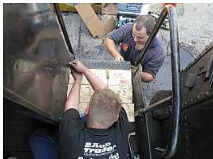
F10 Victor (Bottom) and Andre lay fresh planks on the Driver's entrance side.
