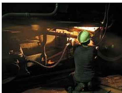
B13 Night shift work on the brakes. Andrew is checking the train-brake vacuum line for leak in the area where it rises from alongside the firebox and runs under the walkway. The flexible pipe in front is the speedometer's signal cable.
