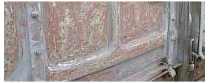
C02 📷 Smooth wire brushed panels. Most of the flaked off paint ended up on Stewart's natty blue overalls.
