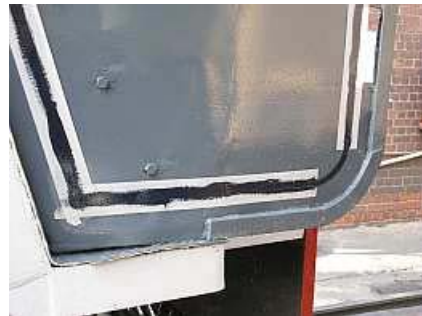
L06 ☞ Locomotive pin striping. Notice that the curved corners are being hand painted.
