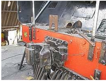
B01 A view of the stripped down brake pipe stand. That mouse-hole leading out to the front deck plate is the pipe aperture.
