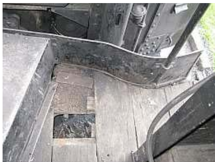
F08 The wobbly floor in the ball room. "Avril's" floor boards are nearly all soft splintery and coming loose from their mountings. This loose plank on the fireman's side was repaired last week.
