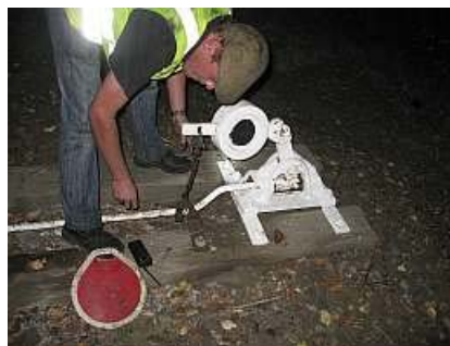
T33 📷 Shaun switches the points over and locks them to guard the occupied sidings. Note the train's tail marker which would be put up in passing as we walk back
