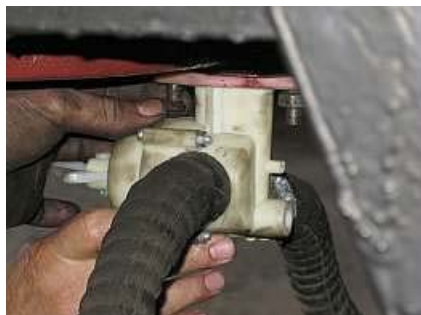
W13 The brake release valve being fitted. The cut down stud is the one to the left and you can just see the new washer being fed over the stud.
