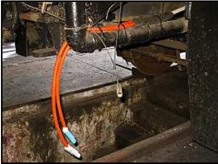
CW04 – Newly installed coach inter-connections strapped to the vacuum brake line. The diagonal cable and the suspended pipe is a cut-cable for opening the coupler.
