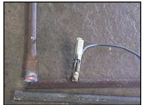
F03 – A lower gate corner, with the weld still cooling and showing the wide welding area at the butted joints.
