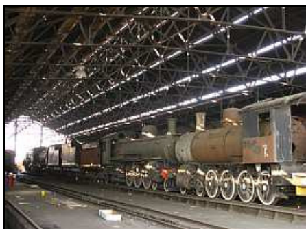
M04 – After some shunting of the Sleeper Coaches being converted to luxury sleepers by Sitemela, the under-cover locomotive restoration line is now visible. Our grand old running shed is one massive structure and the roofing is still in good overall shape.
