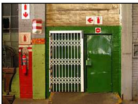
D04 – Refurbished tool store doors. Notice the new fire extinguisher and full set of contemporary and SAR era wide-view-angle fire services signs. This is the number 1 road end of the workshop
