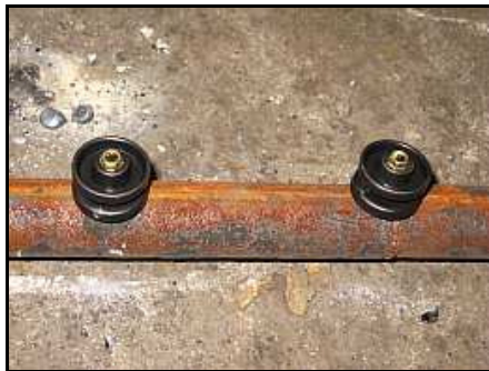
F10 – Two new insulators fitted with modern self-tapping mounting pins.
