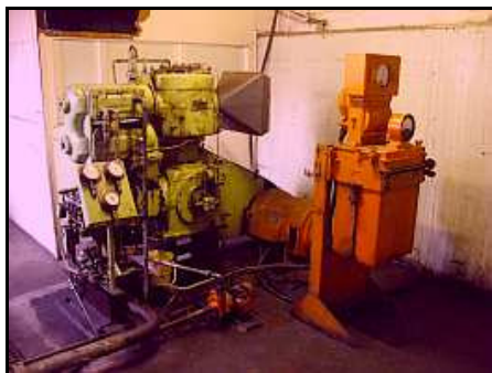
D01 – The old compressor plant. Behind the plant is the office in the corner which has been cleaned and is being converted into a chemicals store.
