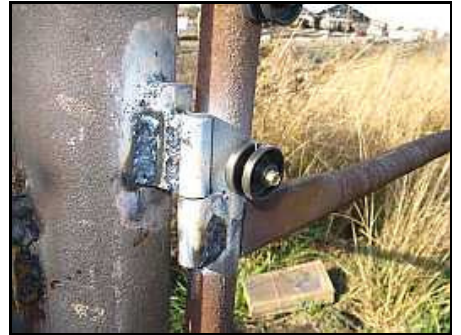
F03 – An assembled upper hinge correctly right at the upper cross rail. The split hinges were mounted in opposite directions so the gate cannot just be lifted off it's hinges
