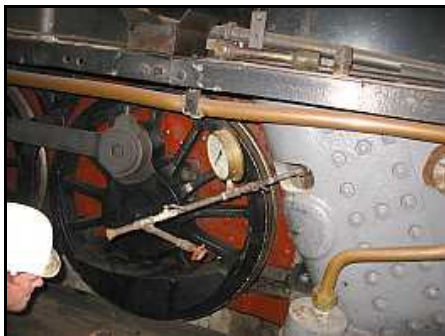
T01 – The vulnerable protruding test coupling screwed into the left wrapper plate’s wash out plug. The downwards pointing pipe is a bleed pipe to provide intake pressure control during the high-pressure low-flow part of the filling process. (As well as being a drain.)
