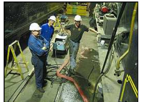
T03 – An important part of boiler hydraulic testing ... the sociable waiting for the boiler to fill up. Left to right – Aiden, Coenie and Shaun, with Patrick and Dawie out of frame, sitting cheerfully on top of the boiler. The pump has just been started in this picture
