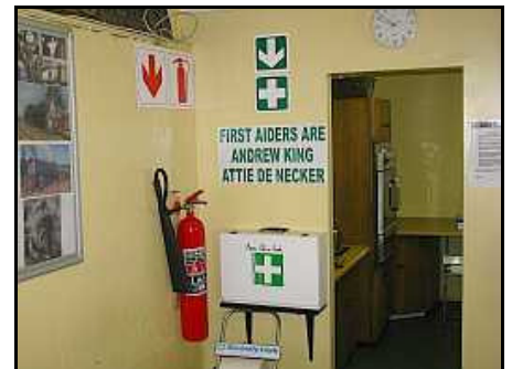
D03 – A safety regulations compliant first aid box and a brand new fire extinguisher, mounted right next to the workshop lounge kitchen door. This area used to be occupied by a rarely used wall mounted TV \ DVD player, which is now in the formal Club House.
