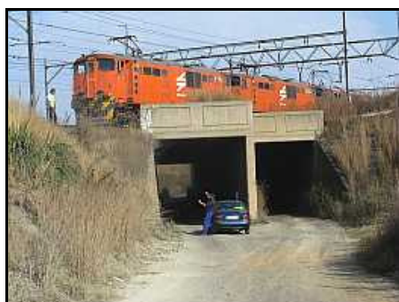
M01 – This is the characteristic double tunnel under the Goods Line on the Reefsteamers approach road. Piet 'Buffels' Steenkamp, who still has many friends and contacts on the railways, chats to the 'unit dryer' as this double headed train of Portland cement bags waits for a green signal.
