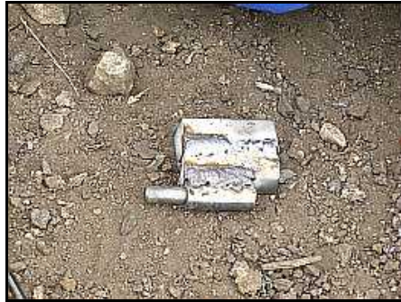
F02 – A fabricated half-hinge has been welded to a spacer block.
