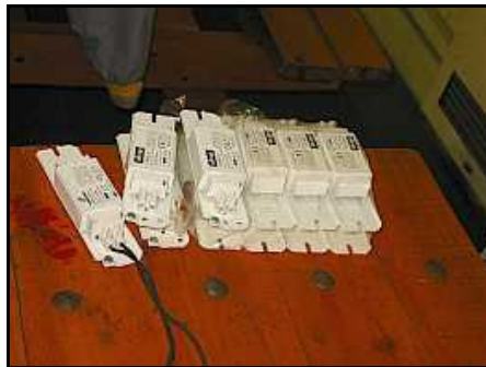
C05 – One down and ten left to go. The wired ballast is a sample, and ten had to be done for the center lighting strip in the coach cabin.
