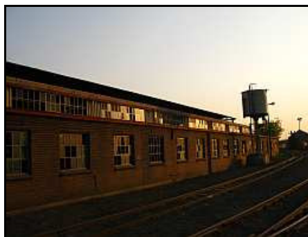
G02 – The Top Shed looks a bit gap toothed in the last light of the day – but look how shiny the new clean windows are in the clearstory rows.
